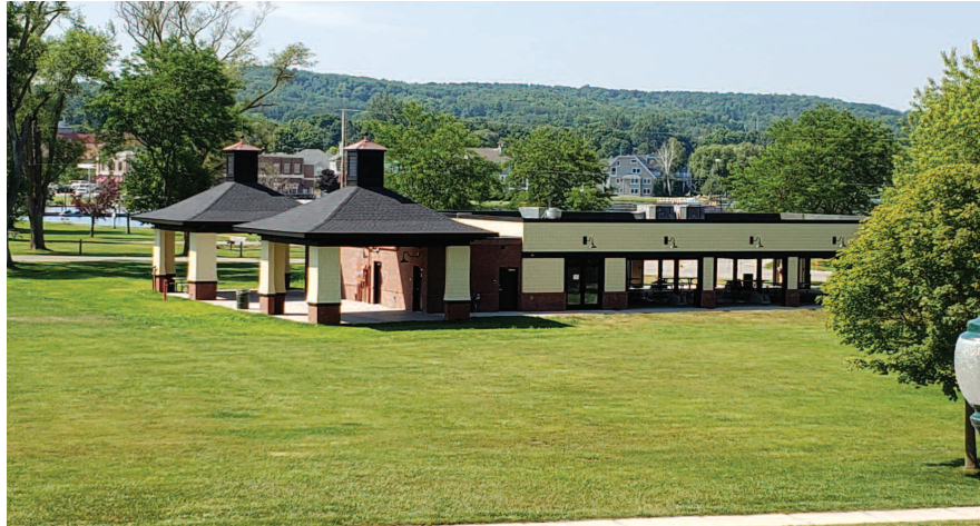
The new Pavilion will be able to be used all year around and in all types of weather.
